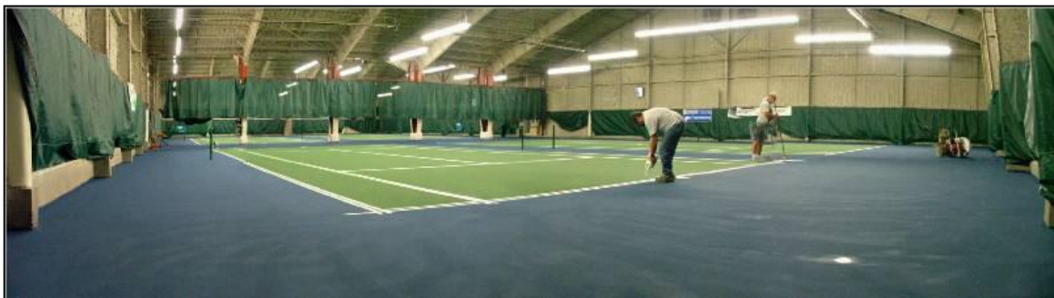
The Tennis Center being resurfaced
